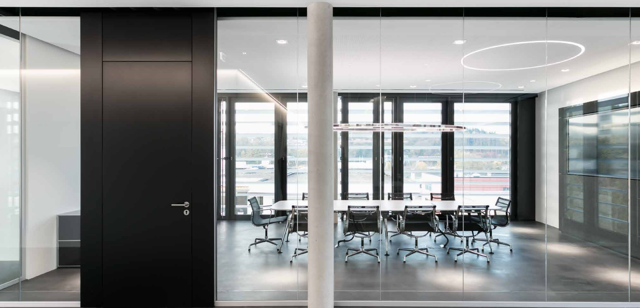
Wooden door element for the conference room with concealed hinges and sound insulation up to 42dB.
