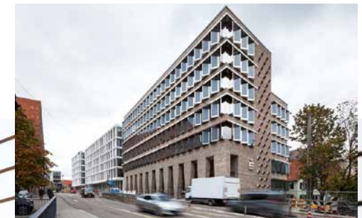
The facade consists of reused bricks.
