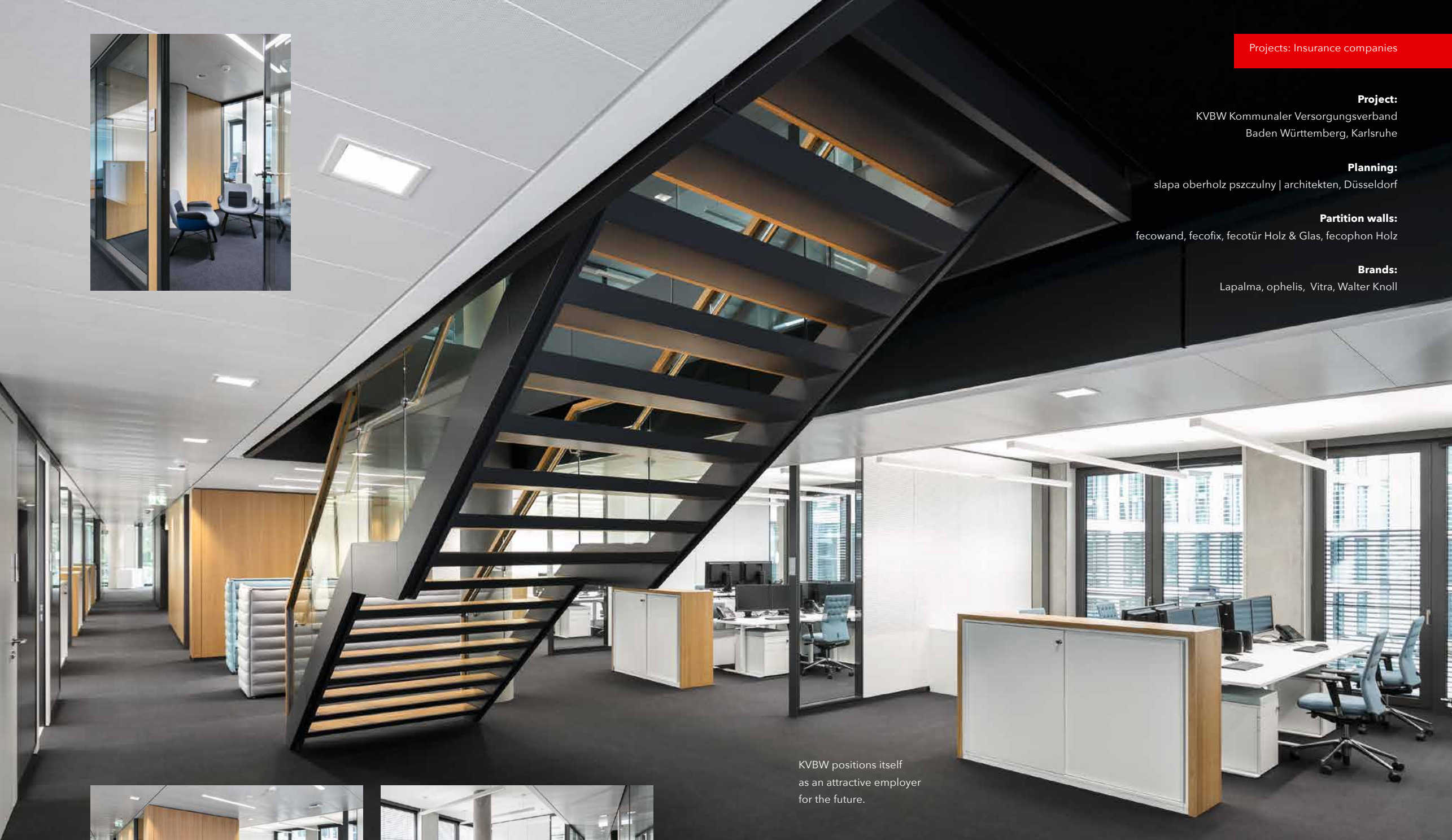
Acoustically-effective fecowand office partition walls structure the office space along the facade. The doors are white, flush-mounted wooden H70 door elements with concealed door frames.
