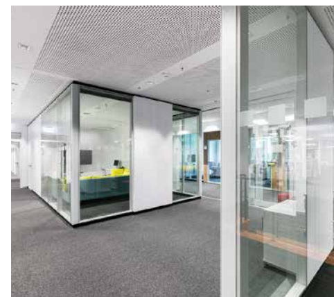
The new office walls have been rendered transparent using the frameless, flush structural double-glazing fecostruct in order to create visual connections to the outside.
