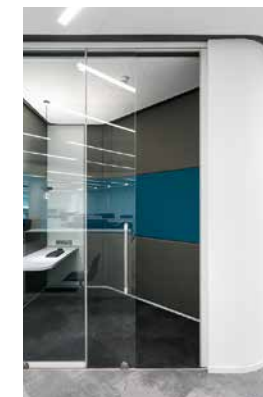
Soundproofed floor-guided glass sliding doors.
